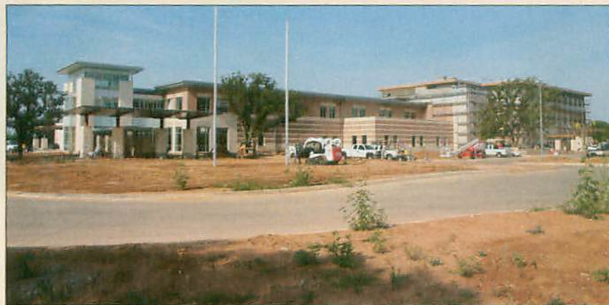
The not-for-profit Doctors' Hospital, Bridgeport, Texas, has taken six years to complete and is scheduled to open by late August.
